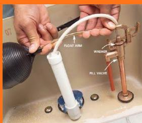
Check to see if the water level is much higher or lower than the line inside the cistern. If so, then you'll need to adjust or replace the fill valve, or the float, both of which regulate the water level in the tank.
