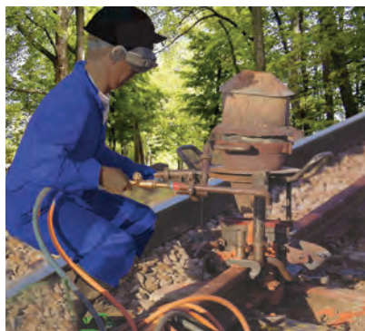
Figure 3.11 Thermit process for joining railway tracks
